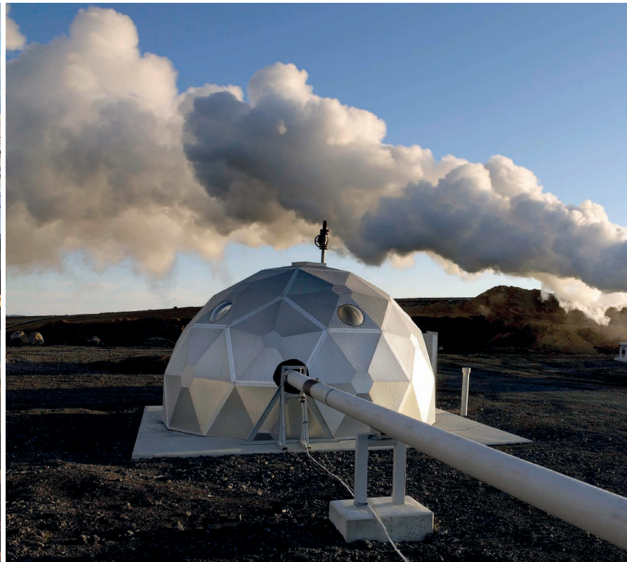
Carbon dioxide injection wells at Hellisheiði geothermal power plant in Iceland.
