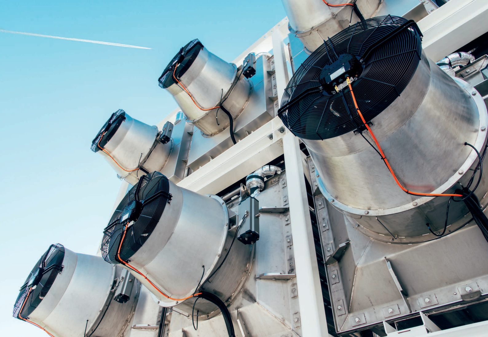
Fans draw ambient air into the Climeworks carbon-dioxide extraction facility near Hinwil, Switzerland.
